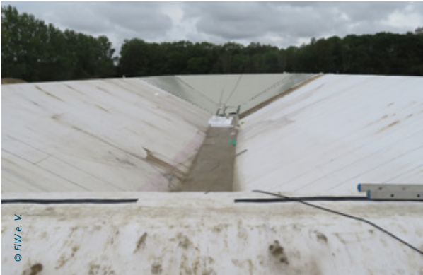
Example of long-term heat storage under construction in Denmark.
